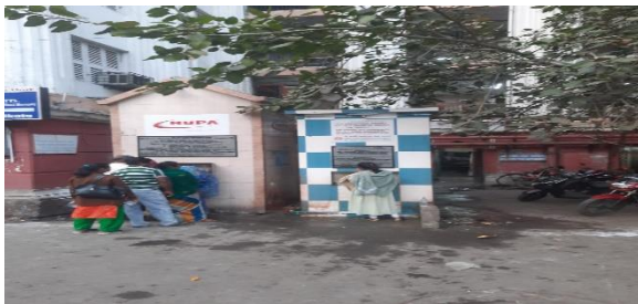
Drinking water facility
