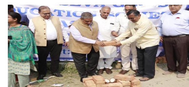
Foundation laid for New Girl's School
