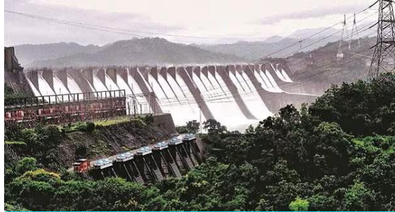
Lower Subansiri Hydro-electric Project, Arunachal Pradesh
