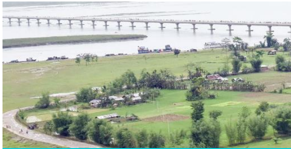
4 Lane Flyover at Mission Chairali, Tezpur, Assam
