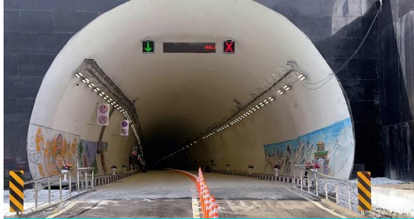
Sela Tunnel, Arunachal Pradesh
