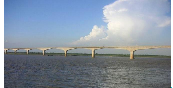
2 Lane Bridge over river Brahmaputra, Assam
