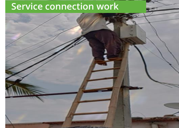
Installation of Conductor Jumpers
