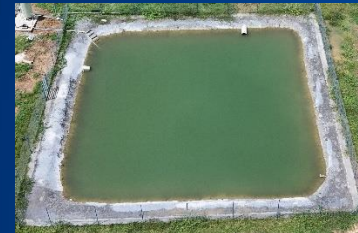
Rainwater collection pond at Oragadam site supports 70% freshwater needs for domestic use
