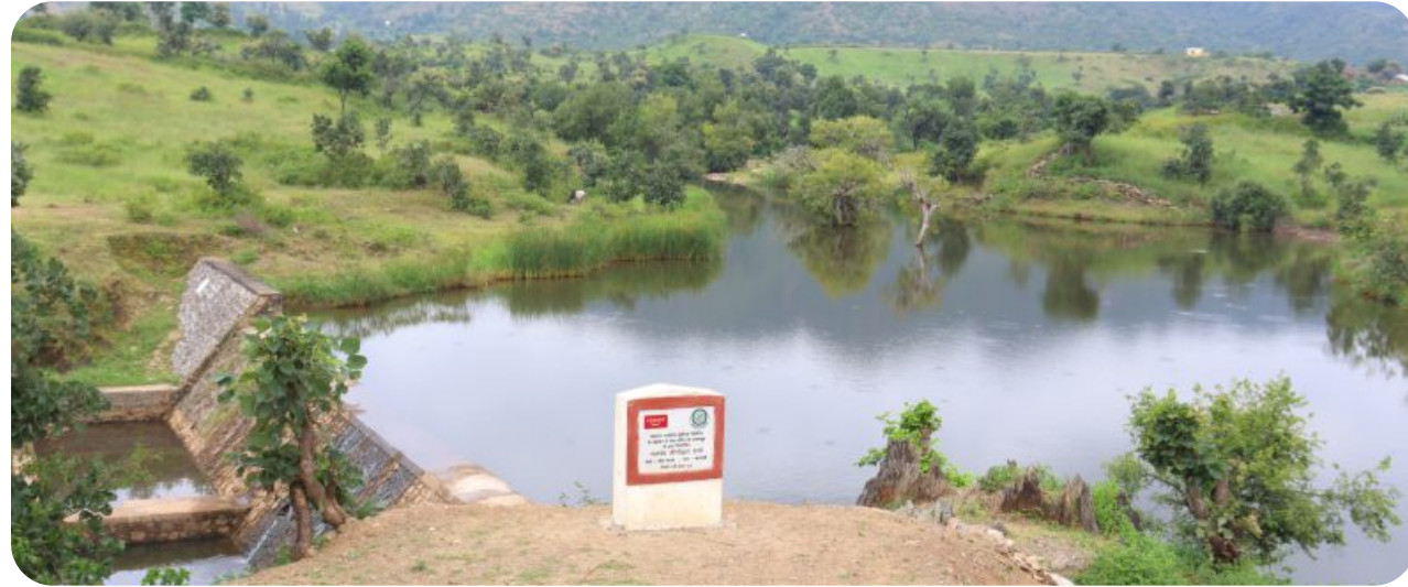
Anicut Restoration, Kaliwas Village, Rajasthan
