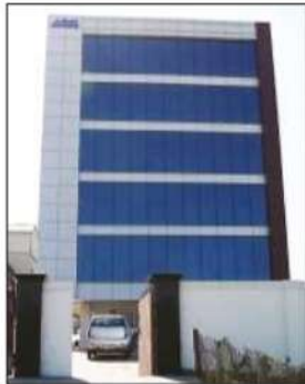
55,000 Sq.ft Facility in IDA Mallapur, Hyderabad Unit-I
