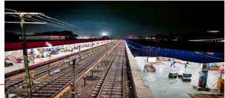
NBQ-GLPT-KYQ Doubling Project (Assam).
