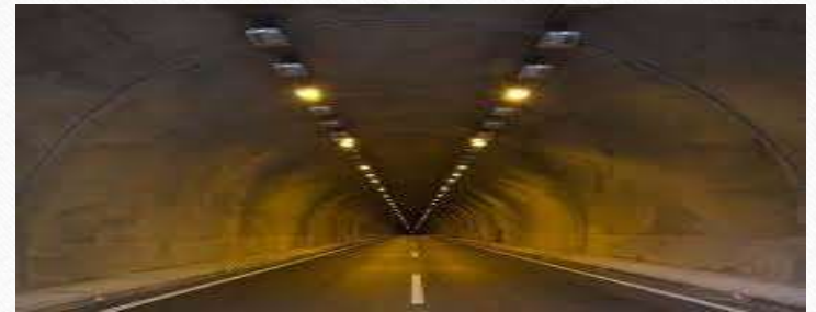
Construction of single line BG cut & cover tunnels from in between stations Kawnpui to Sairang including counterfort retaining wall on pile foundation & protection work along with all other ancillary works.
