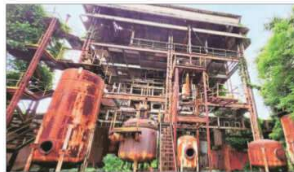
The toxic waste is being shifted in 12 sealed container trucks to Pithampur industrial area, 250 km away from Bhopal
