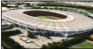
Roof Structure Ropes
