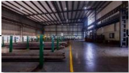
Covered Raw Material Yard
