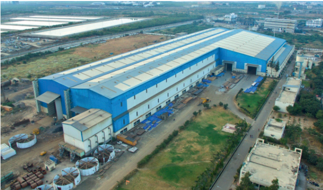
Manufacturing Shops at Dahej, Gujarat, India
