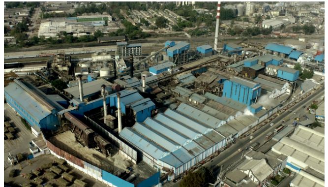
Sugar Mill and Ethanol Plant at Yamunanagar, Haryana, India
