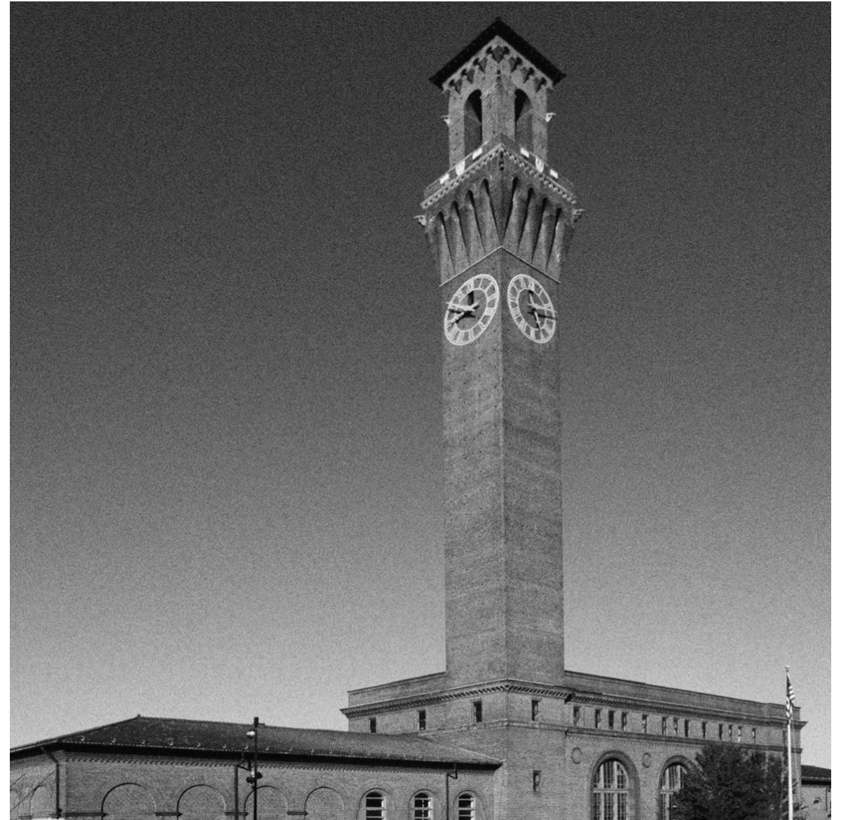
Waterbury Clock Tower
