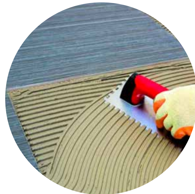
Tile and Stone Installations
