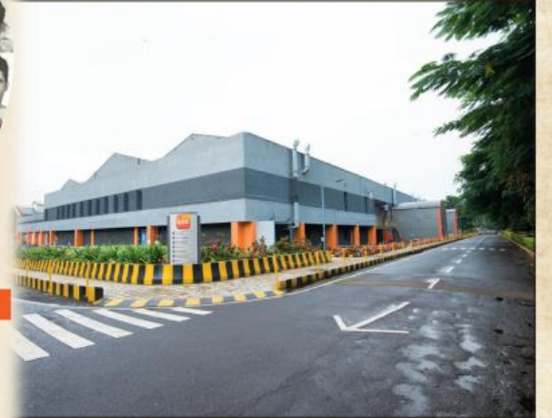
▲ GSK India's present-day manufacturing factory located in Nashik, Maharashtra
