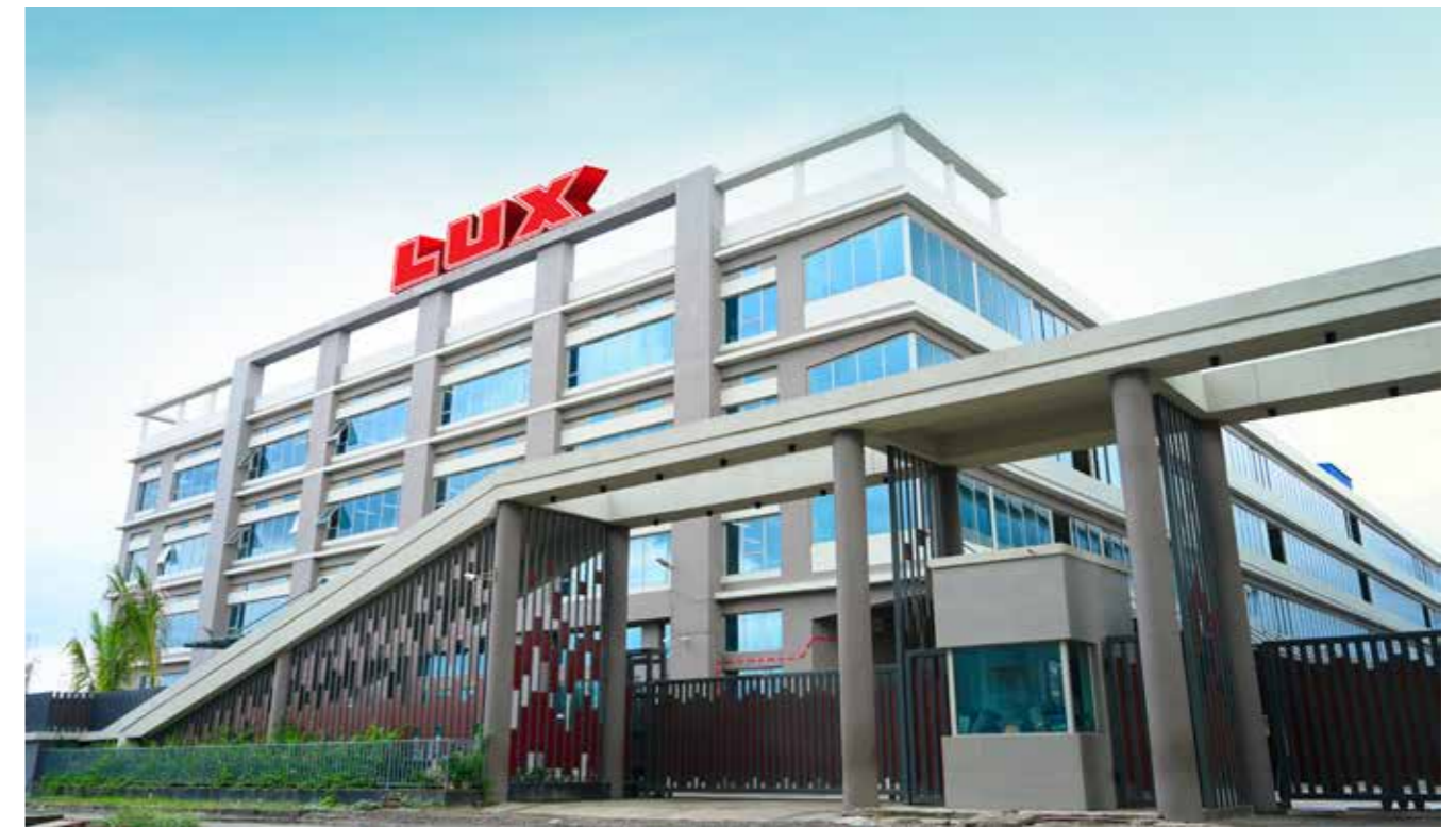
Jagadishpur, Hosier Park Facility
