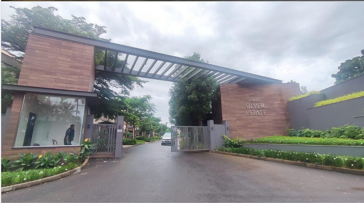
Sobha Silver Estate Thrissur
