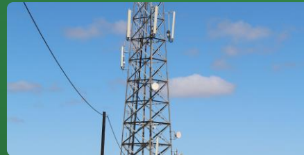
Telecom Tower Structure
