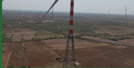
Windmill Lattice Tower
