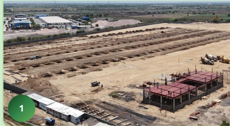
Land parcel at the Matar site
