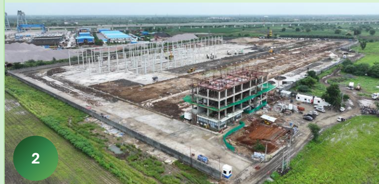
Site preparation & civil works started at the new site
