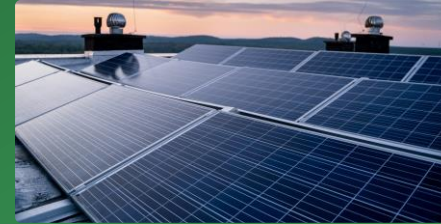
Solar Rooftop Installation
