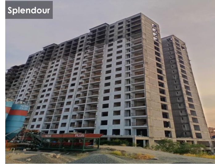
Project Status as on Mar2024
