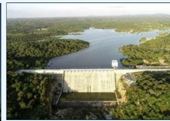
500 Mcft Gravity Dam, Karnataka
