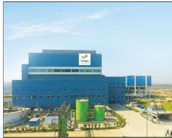
24 MW Waste to Energy Plant, Delhi
