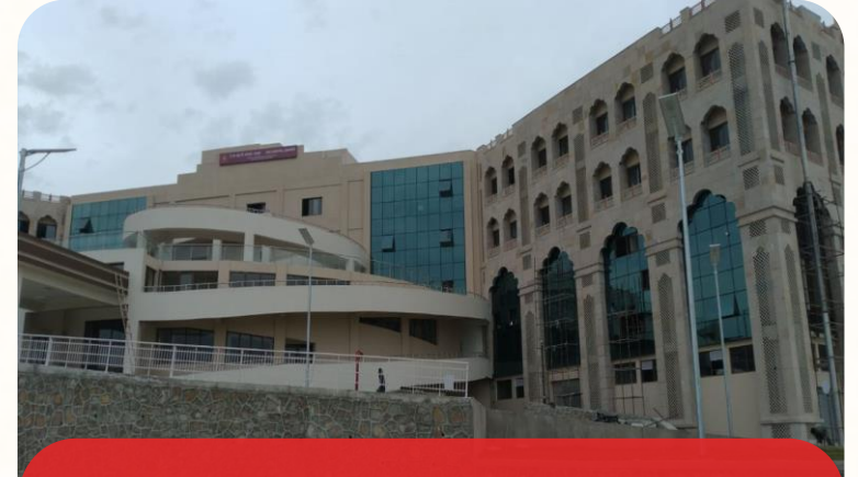
Hospital Project In Udaipur Rajasthan
