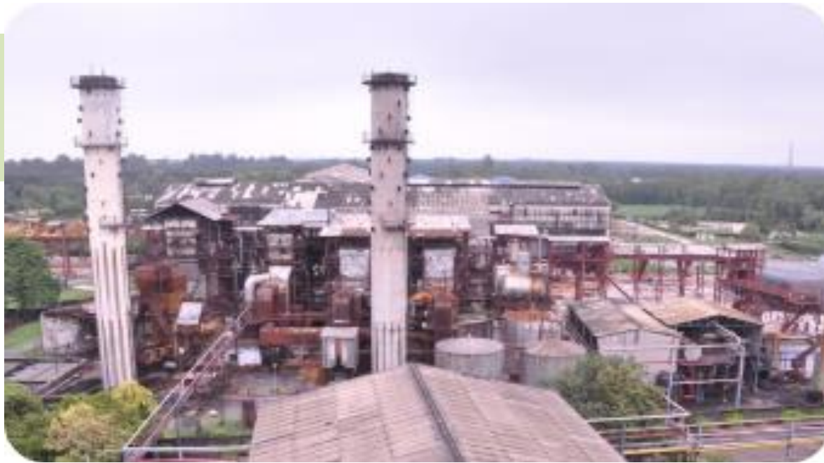
Sugar plant overview
