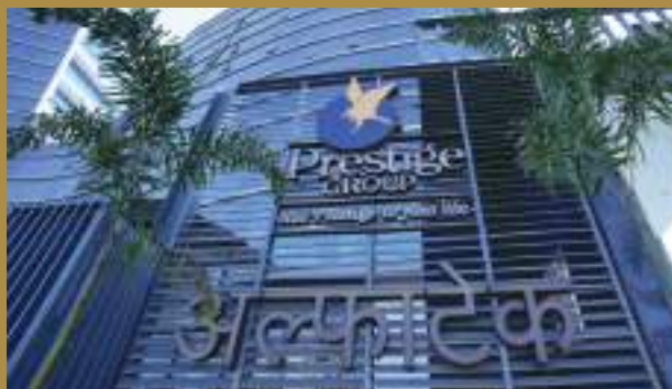
Prestige AlphaTech, Kharadi, Pune
