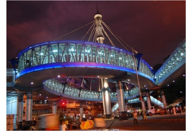
Grant road Skywalk
