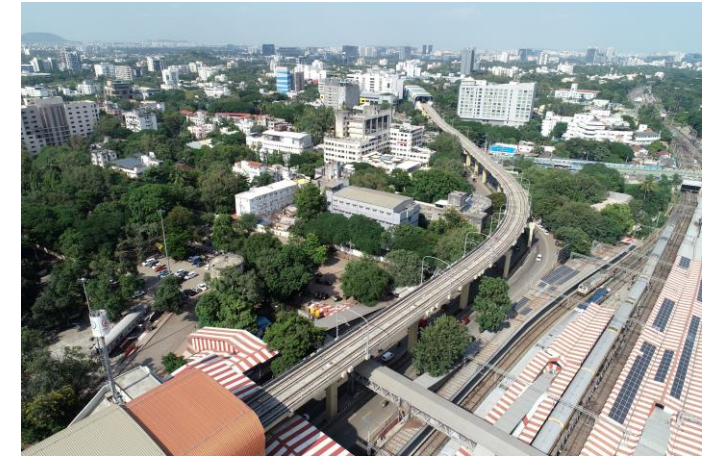
Pune Elevated Metro
