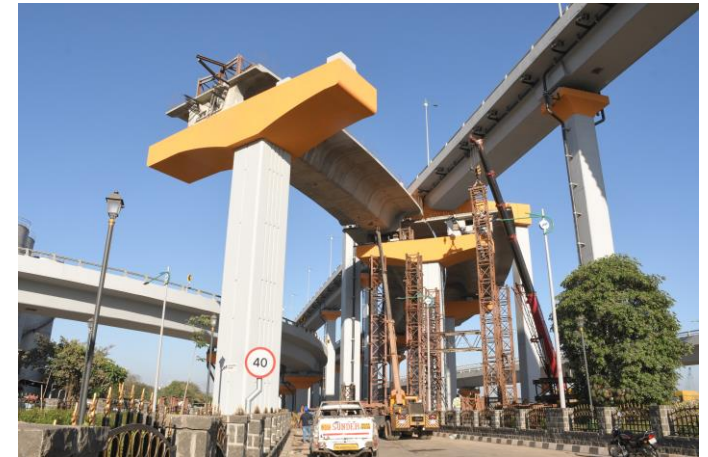
Sewri Worli Elevated
