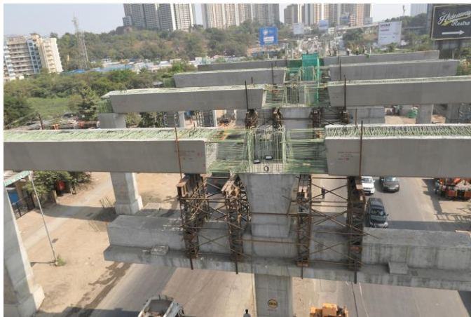
Mumbai Metro Line 4A
