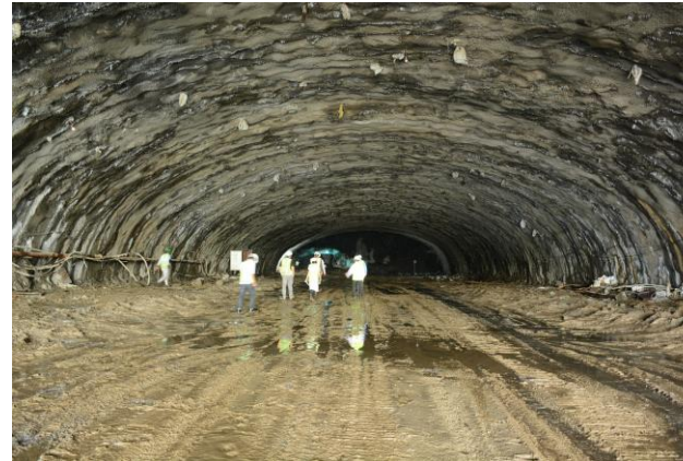
Vadodara Mumbai Expressway, IRCON
