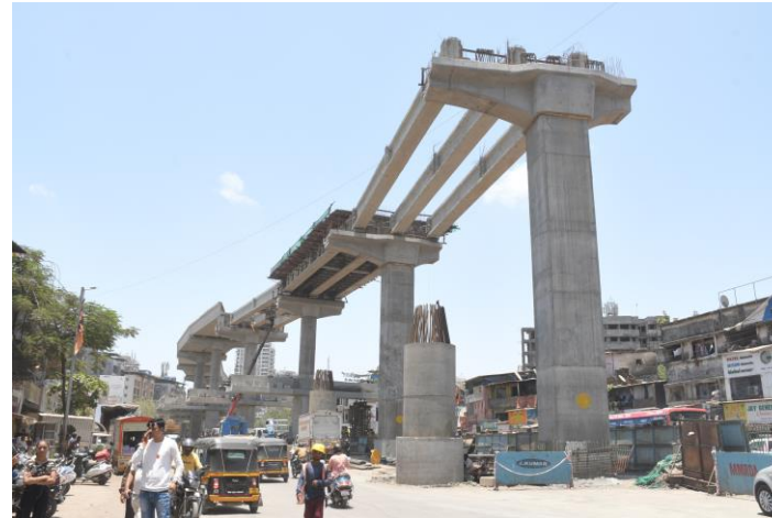
Mumbai Metro Line 9
