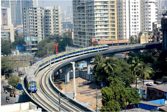
Mumbai Metro Line 2A
