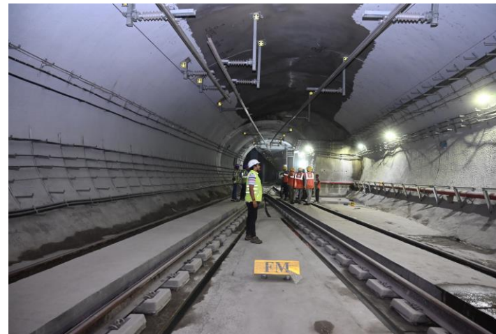
Mumbai Metro Line 7A
