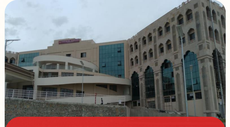
Hospital Project In Udaipur Rajasthan
