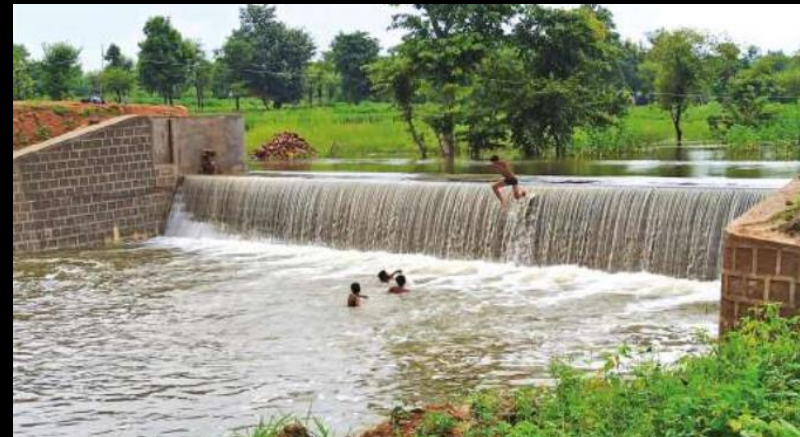
Recharging Ground Water Table
