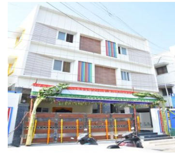
New Building with area of 5600 sq ft for school for special kids
