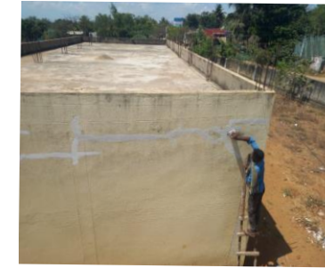
Repaired existing government run school building
