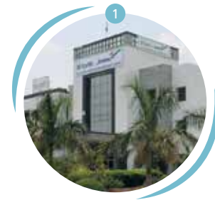
Fortis OP Jindal Hospital & Research Centre, Raigarh
