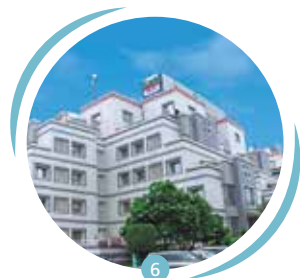
Fortis Ft. Lt. Rajan Dhall Hospital, Vasant Kunj, New Delhi
