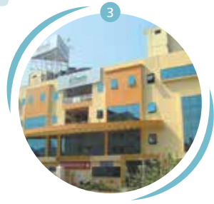
Fortis Hospital, Nagarbhavi, Bengaluru
