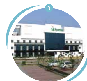
Fortis Hospital, Chandigarh Road, Ludhiana
