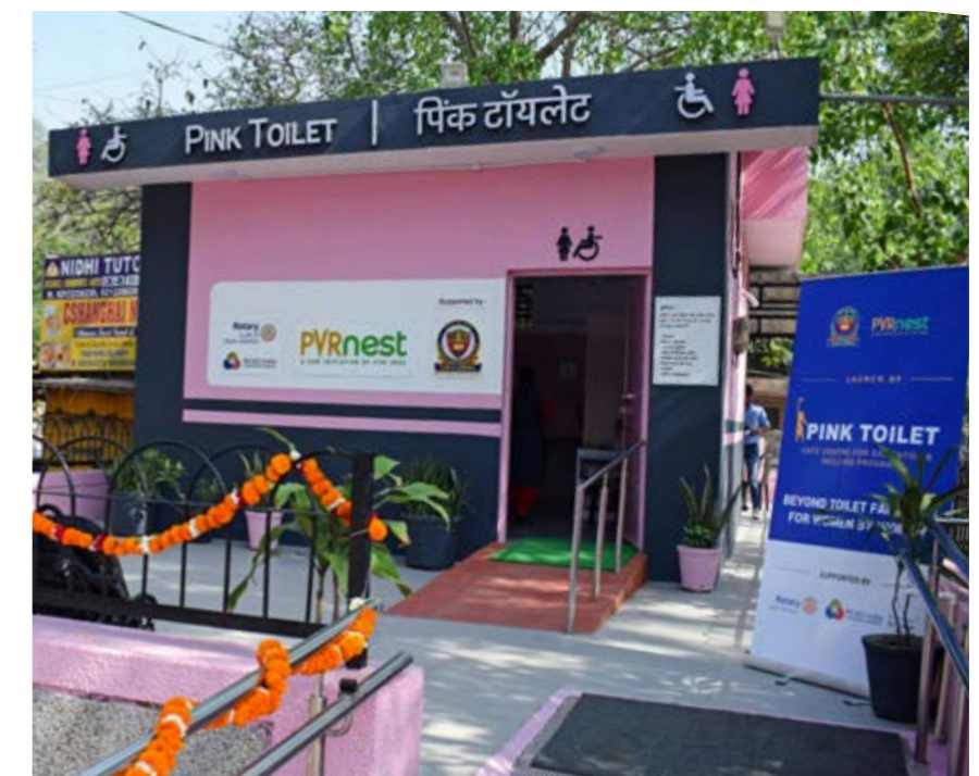
» Beyond Toilet Facilities
