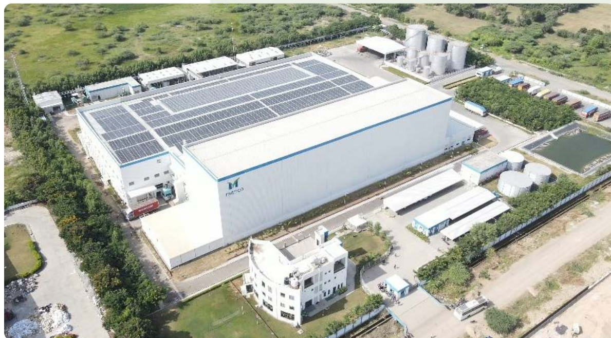
1 MegaWatt Renewable Energy generation @ Sanand unit
