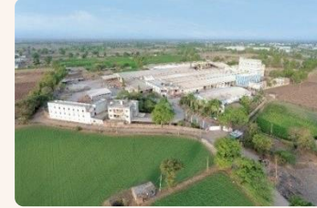
AGL Idar Plant (Floor Tiles)
