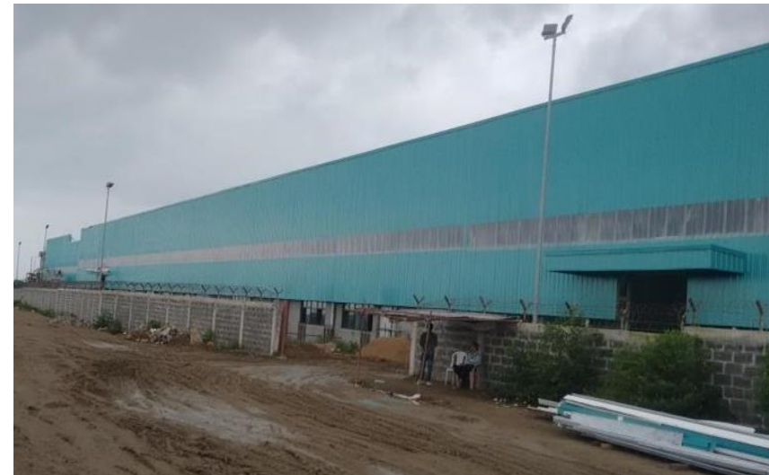
MRF - Factory Warehouse
