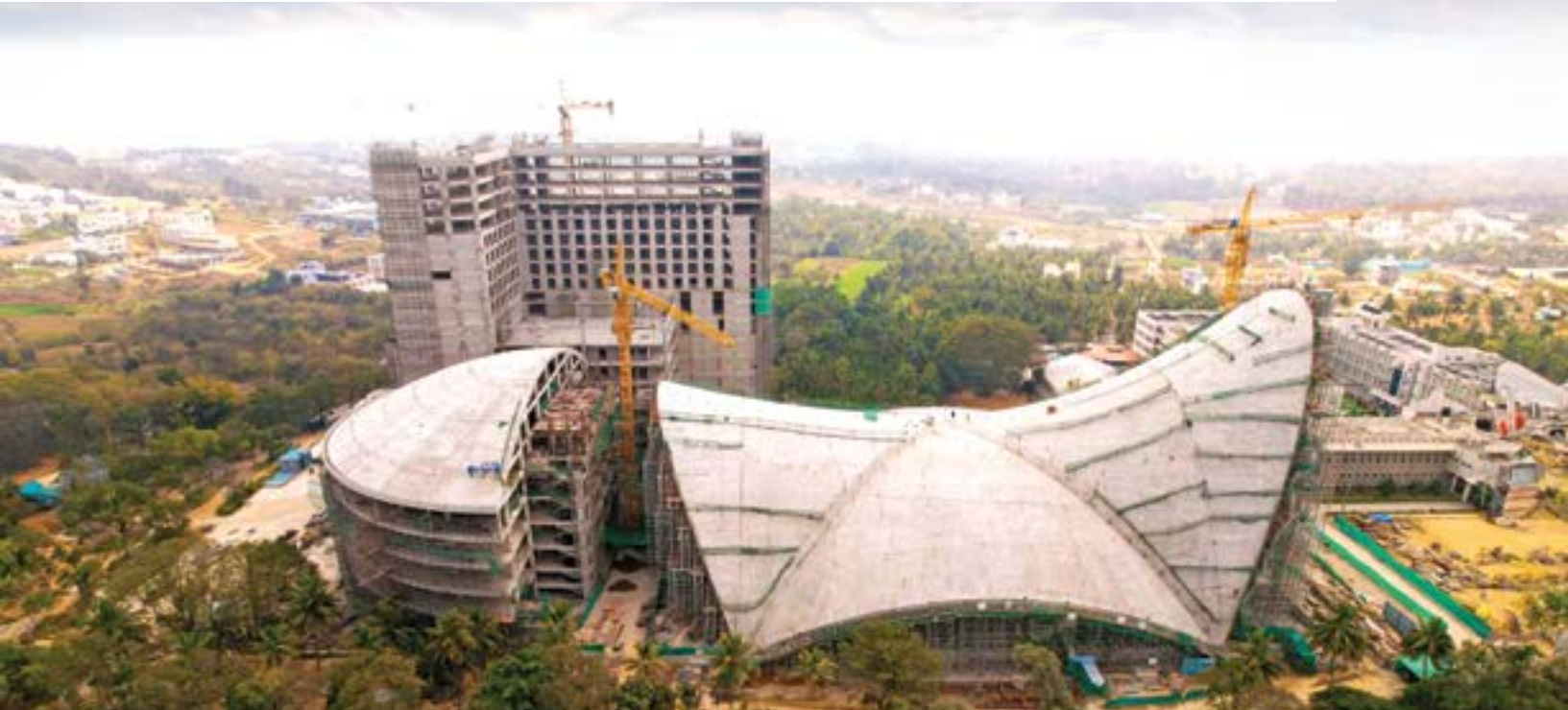
World's largest thin shell RC structure (JSVK Convention Center, Bengaluru)
