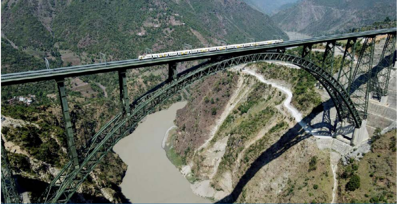
Chenab Bridge High Speed Test Run
