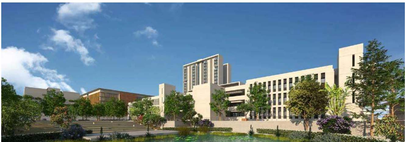
RBI Green Field Data Centre in Bhubaneswar
