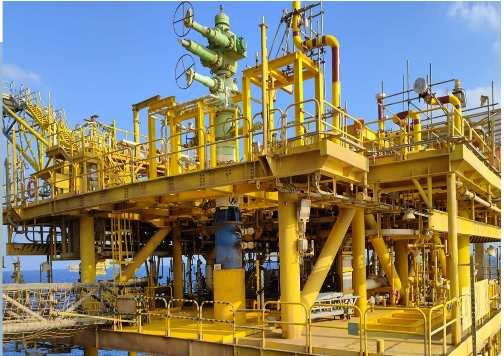
CRPO 75 Arbi 8 Refurbishment Project
