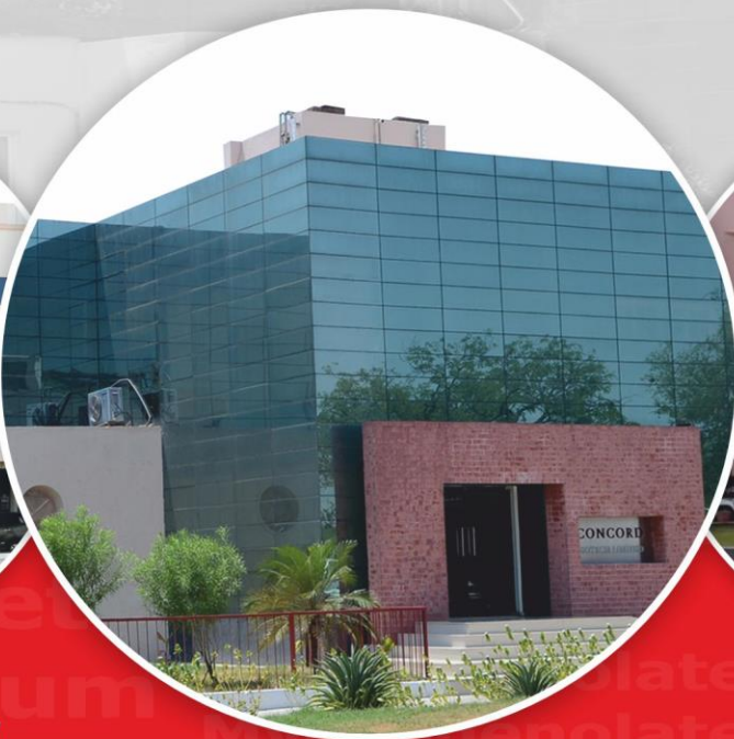
API Facility Dholka, Ahmedabad, India
