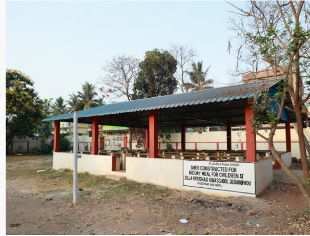
Shed constructed for midday meal for children at jilla parishad high school – Ippanapadu.
