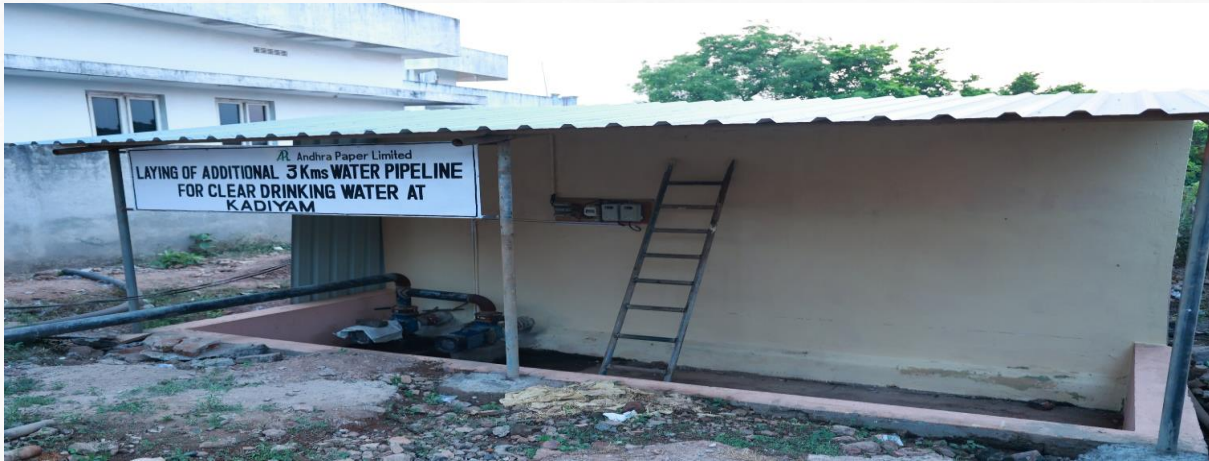
Construction of additional Water Pipelines for clean drinking water at Kadiyam
