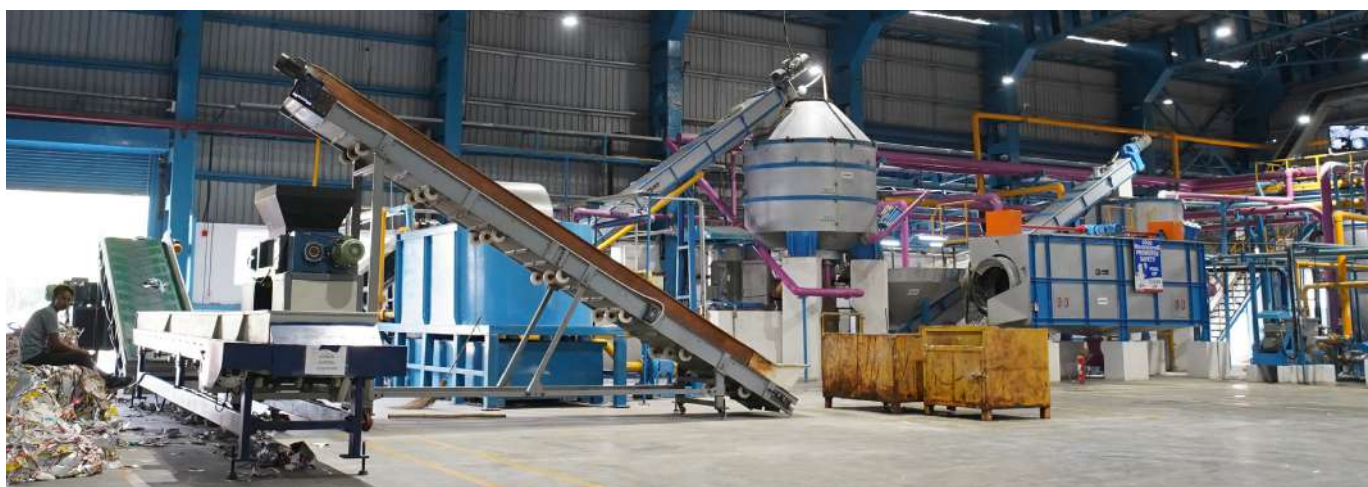
UFlex's aseptic recycling plant at Malanpur, MP, India
