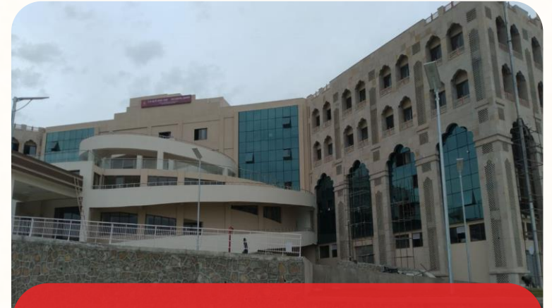
Hospital Project In Udaipur Rajasthan
