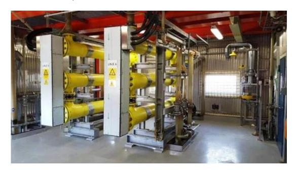
2. Successfully designed, manufactured and supplied 24 Pulse DC Rectifier for Electrolysis application (Hydrogenation / Electro Chlorination) for various Power plants and Oil Refinery with 77mm and 100mm devices.
