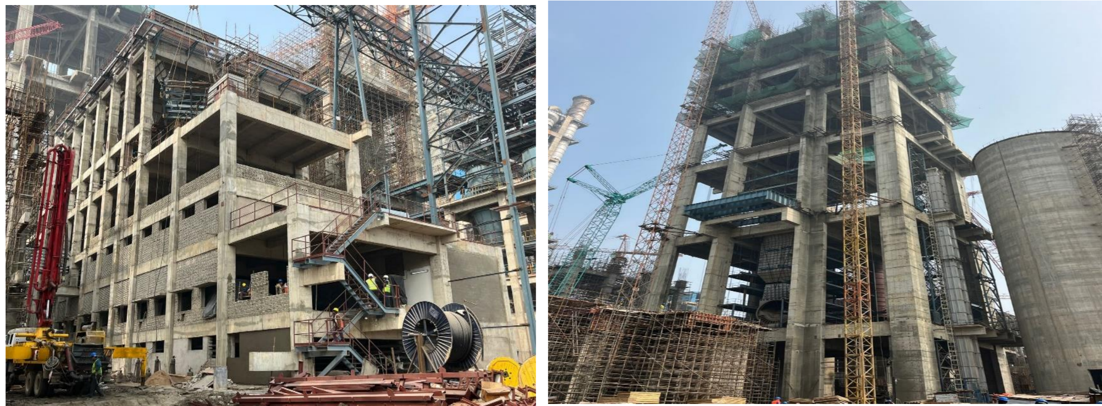
Panna Line-II- RM Bag House , Pre Heater building & Silo
