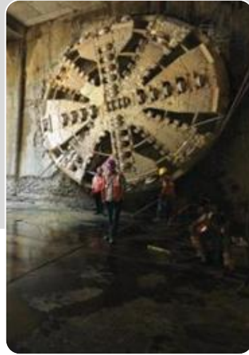
16 Tunnel Boring Machines (TBMs) +4 Pending Delivery
