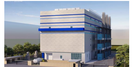
DATA CENTER BUILDING
