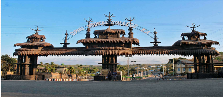
Construction Of Assam Hills Medical College & Research Institute, Diphu, Karbi Anglong.
