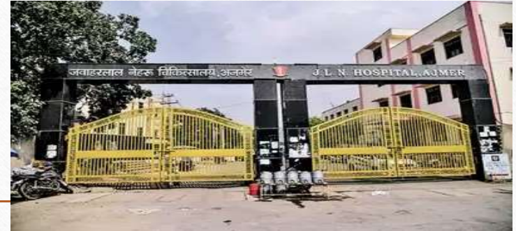
Construction of Medicine Block at JLN Hospital, Ajmer, Rajasthan.
