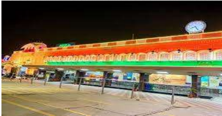
Major upgration of Gandhinagar (Jaipur) Railway Station of Jaipur Division of North Western Railway through EPC.
