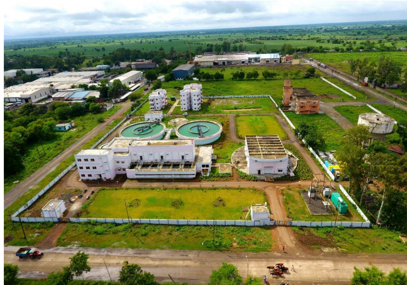
Industrial Water Treatment Plant, Dewas, Madhya Pradesh
