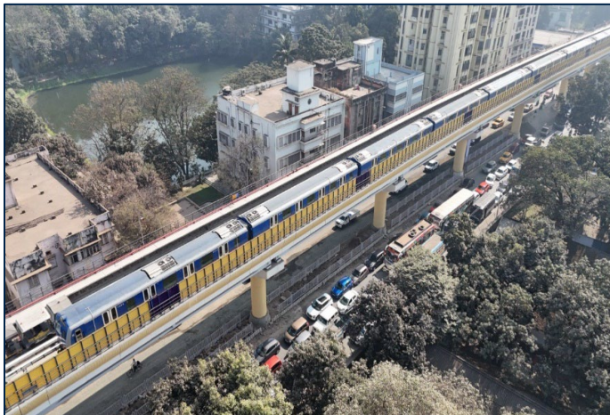
Metro Rail Bridge- Majerhat
