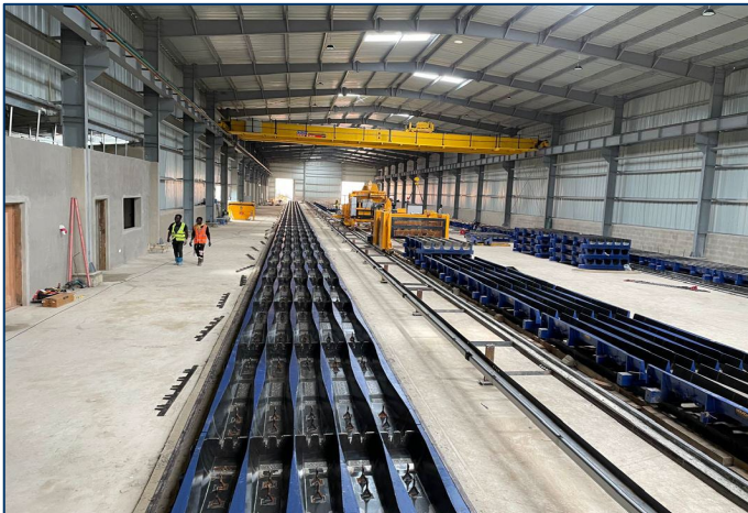
Concrete Sleeper Factory- Ghana
