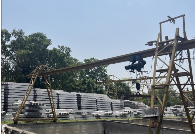
Concrete Sleeper Factory- Panagarh
