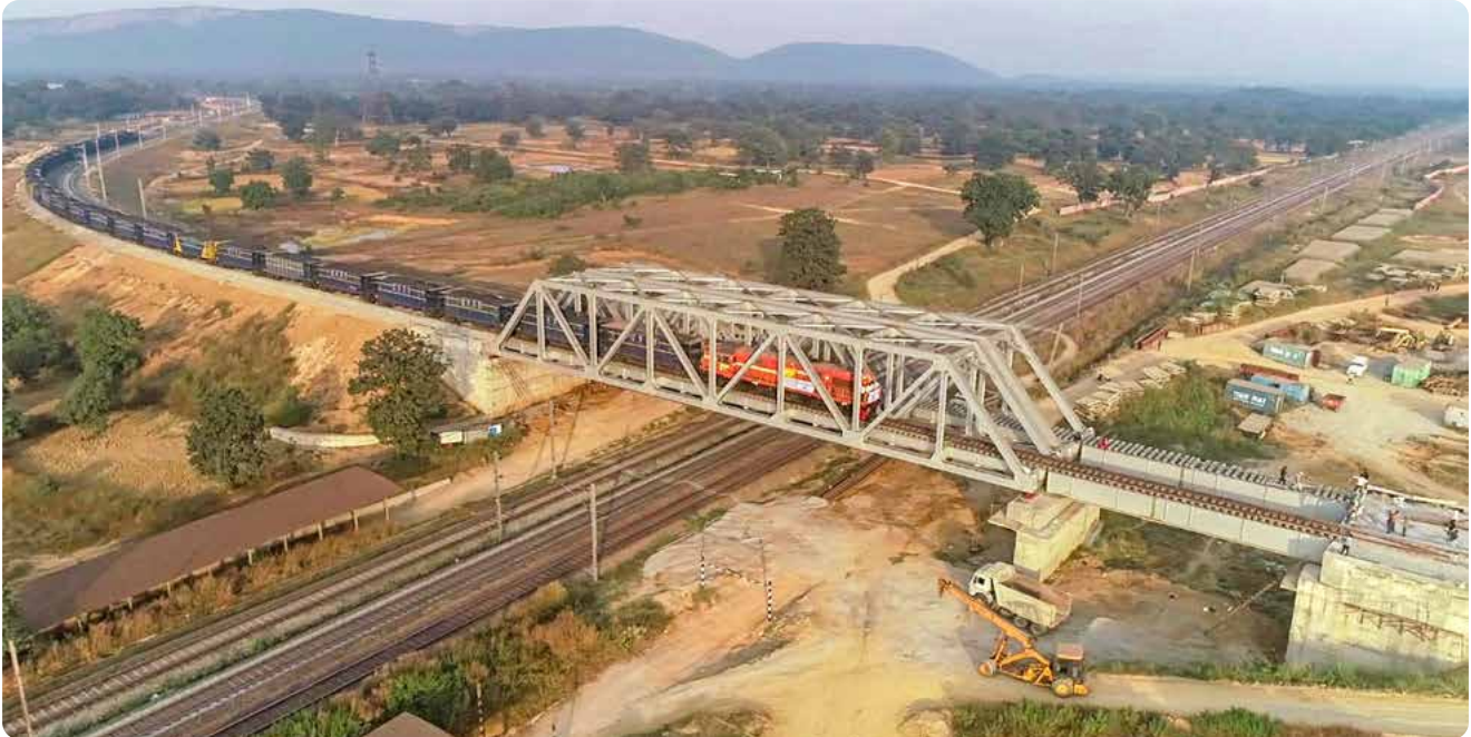
● Consultancy of a rail siding at NTPC-Tarapalli
