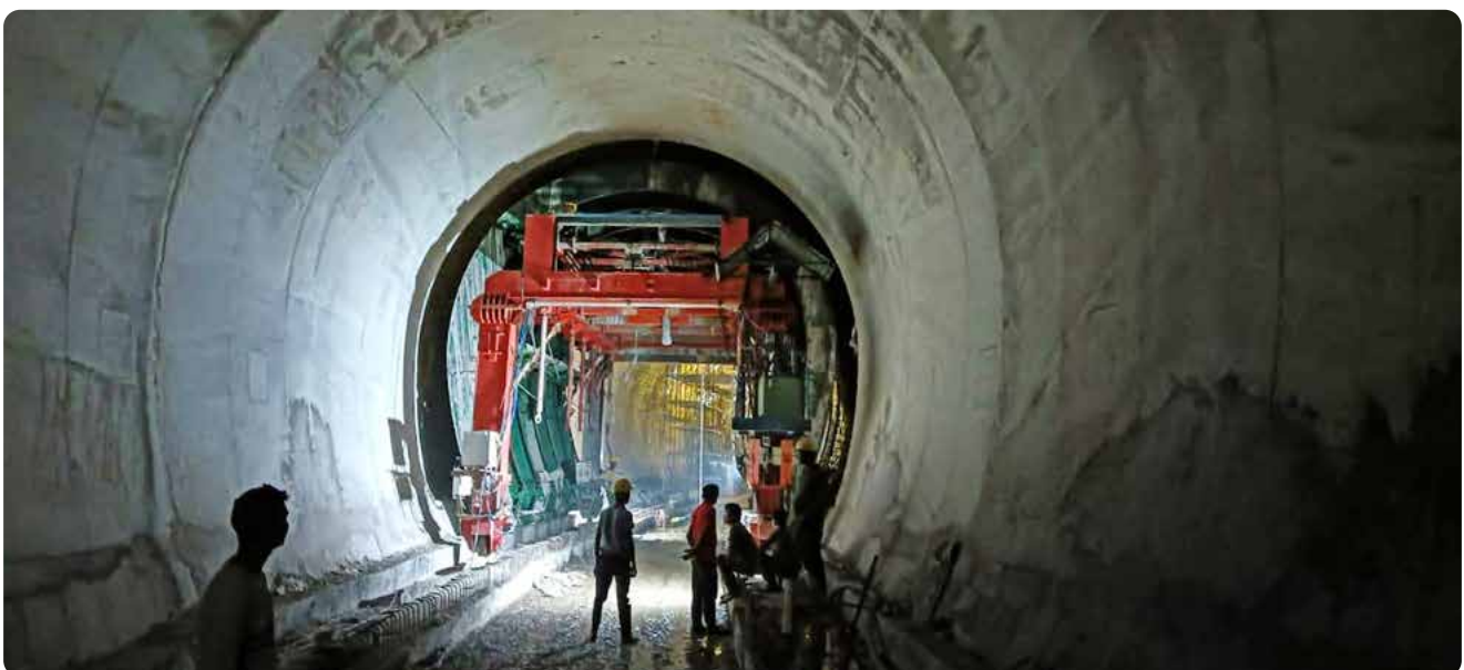
▶ T-1 tunnel under construction at the Manabar-Jarati-Maligura section in Odisha
