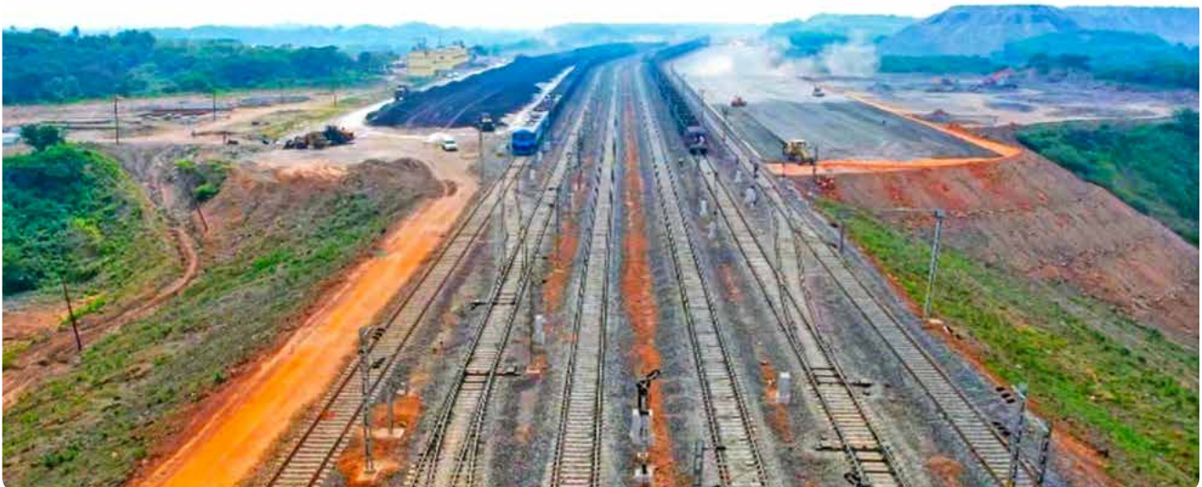
▶ New y-curve, a first-mile connectivity project of CIL between Brajrajnagar & Lajkura station of South Eastern Railway on the Howrah-Mumbai trunk route in Odisha
