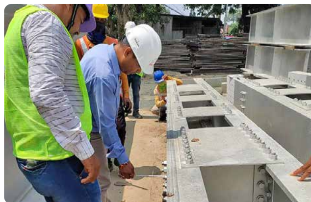
Third Party Inspection for rail equipment
