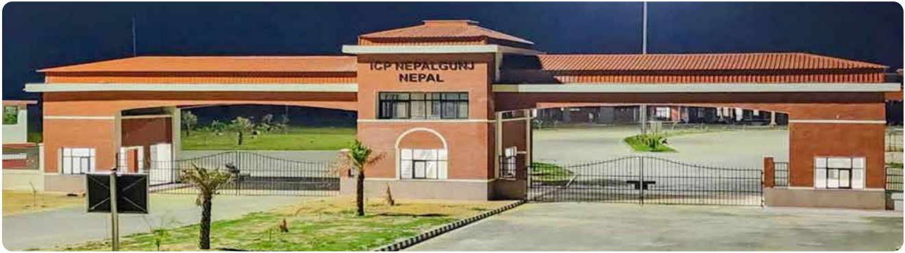
► Project Management Consultancy for the Nepalgunj Integrated Check Post, Nepal
