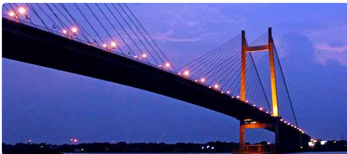
▶ Repair and rehabilitation of the 2 nd Hooghly Bridge (Vidyasagar Setu) in Kolkata
