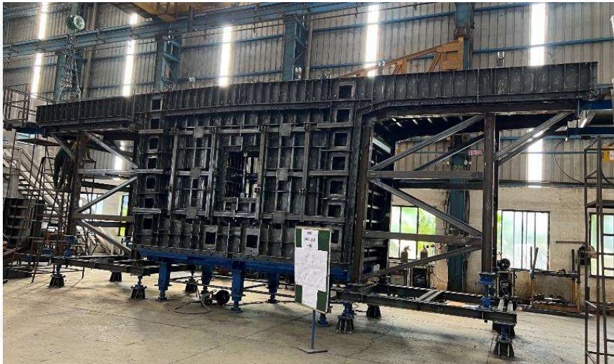
Pier Head Segment
