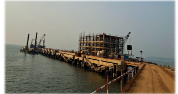
LPG construction at Jaigarh Port
