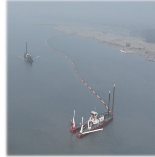
Dredging work underway at Jatadhar
