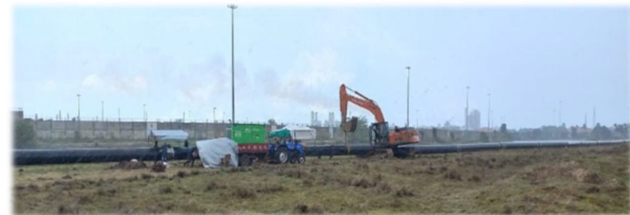
Setting up slurry pipeline
