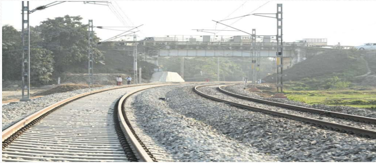
Construction of sub-structure and super-structure on pile foundation of major bridges in connection with double line work of New Bongagaon-Agthori doubling project.
