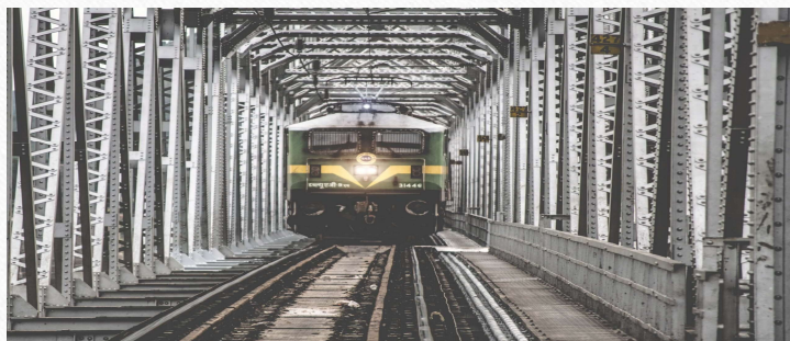
New BG Railway line project.
